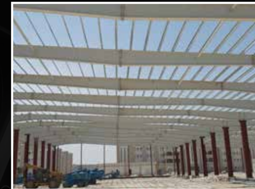
Steel Fabrication and Installation
