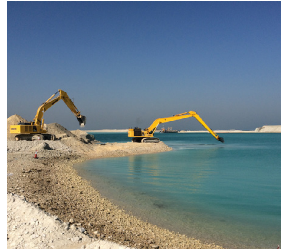
Excavation of Swimmable Area
